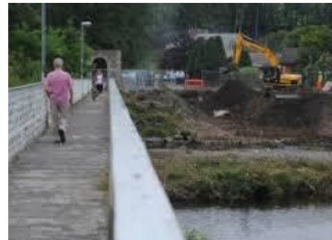
Flood prevention scheme underway
